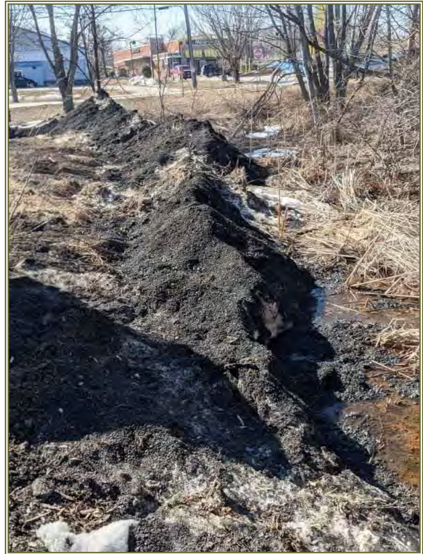
Drainage swale on west side of building with snow bank from plowed parking lot looking south
