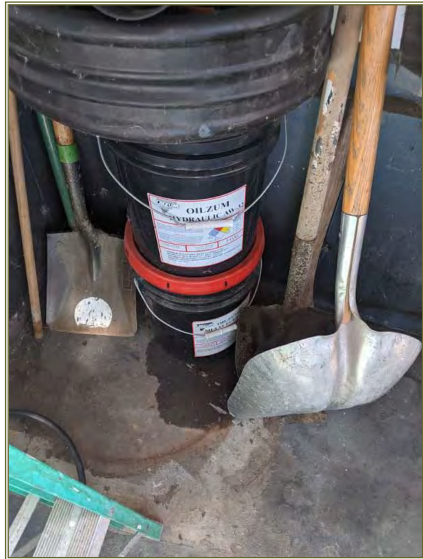
Floor staining from hydraulic oil
