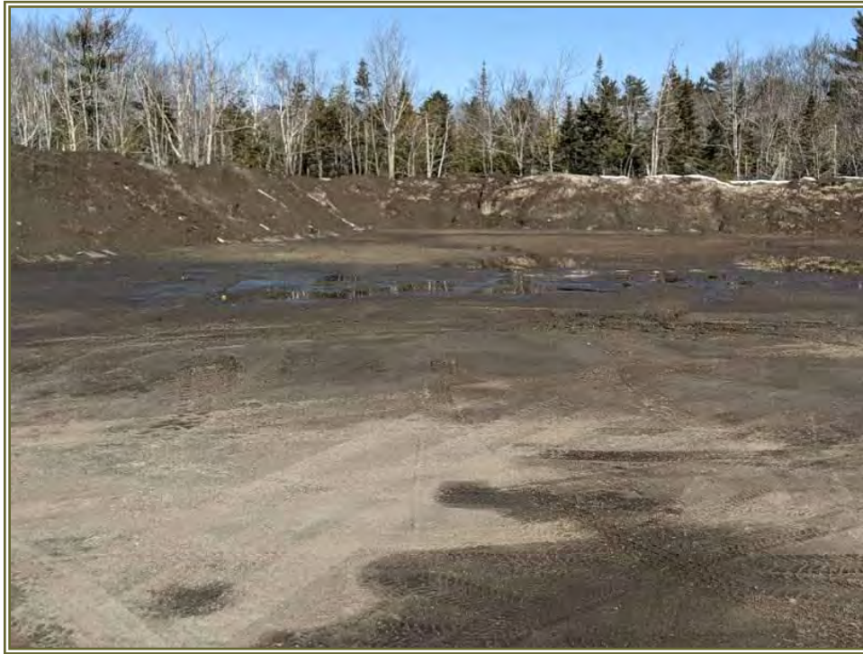
Snow piles located north of Fire Station building looking northwest
