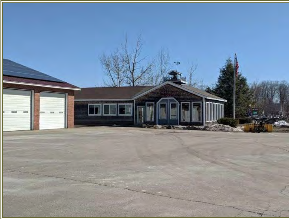
West side of Museum building located east of Fire Station building looking northeast
