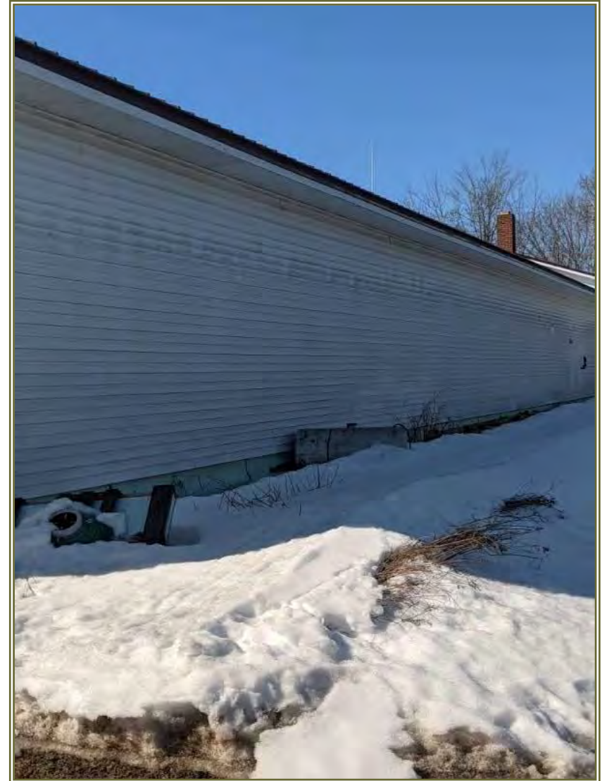
North wall of Fire Station building with water tank near center
