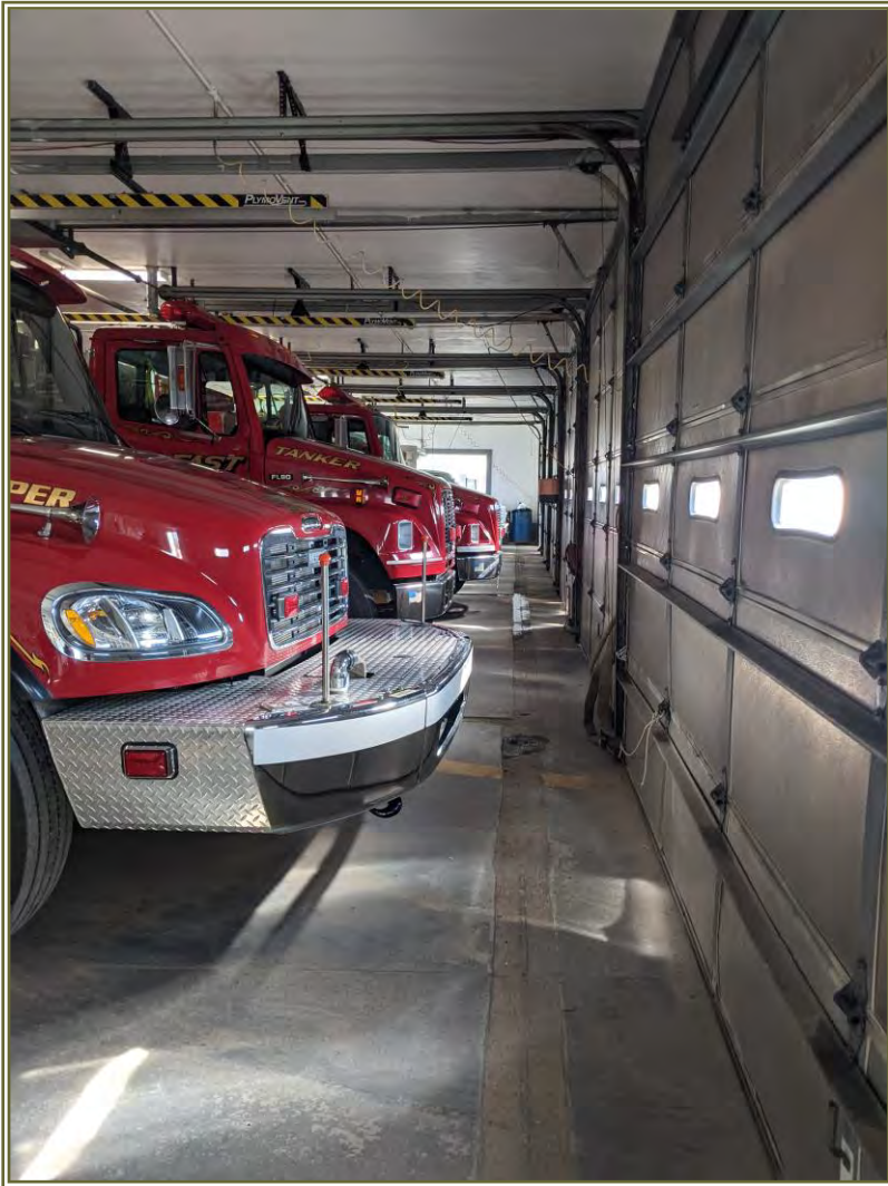
Scarified trough inside garage bays for deterring outside stormwater
