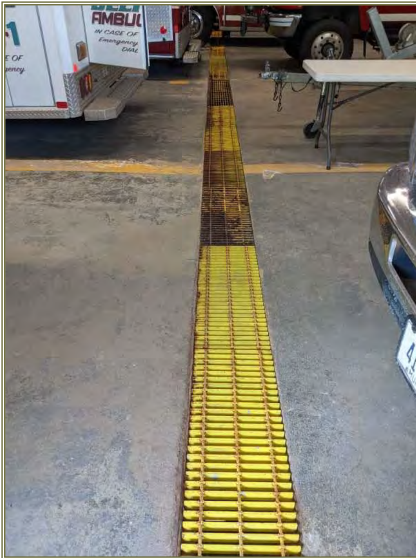
Floor trench that runs east-west through the original fire station building
