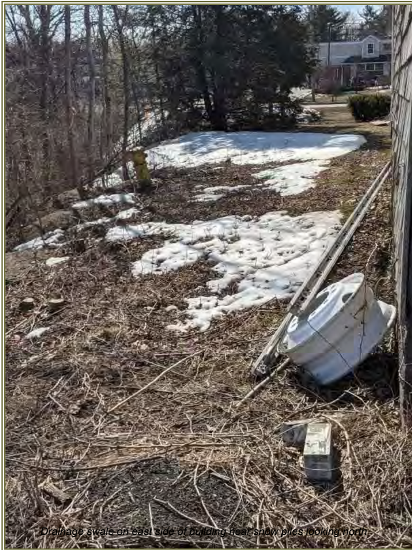
Miscellaneous debris along east side of Fire Station Building looking south
