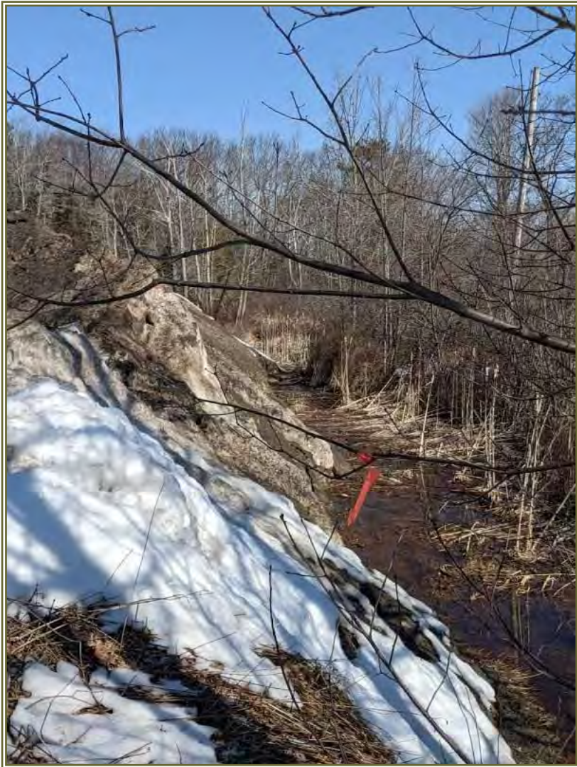
Drainage swale on east side of building near snow piles looking north
