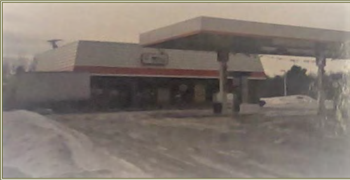
Former CN Brown, Big Apple service station at 268 Main Street, Map 012, Lot 40, photograph source tax assessor
