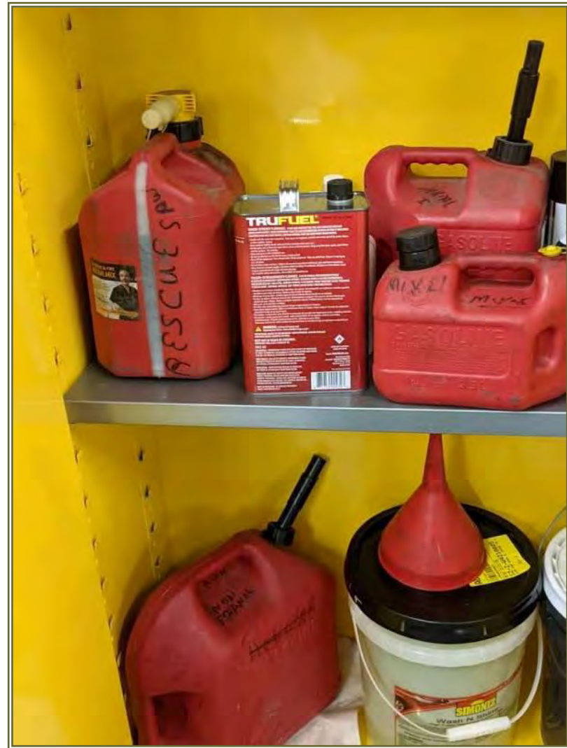
Gasoline and oil stored inside the flammable cabinet
