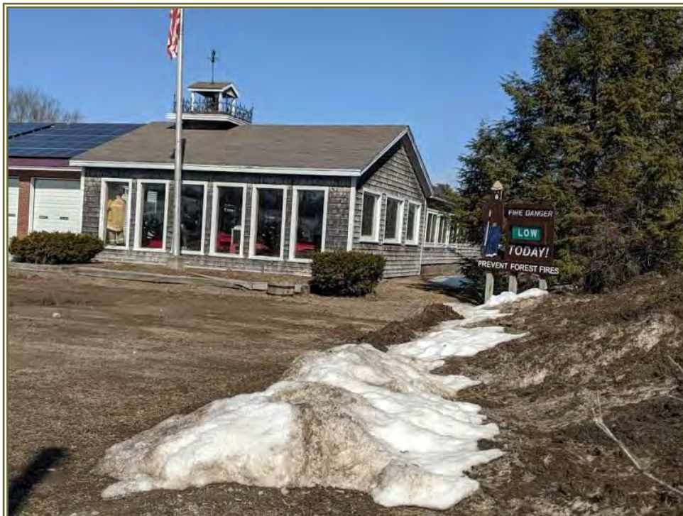
South and east side of Museum building looking northwest
