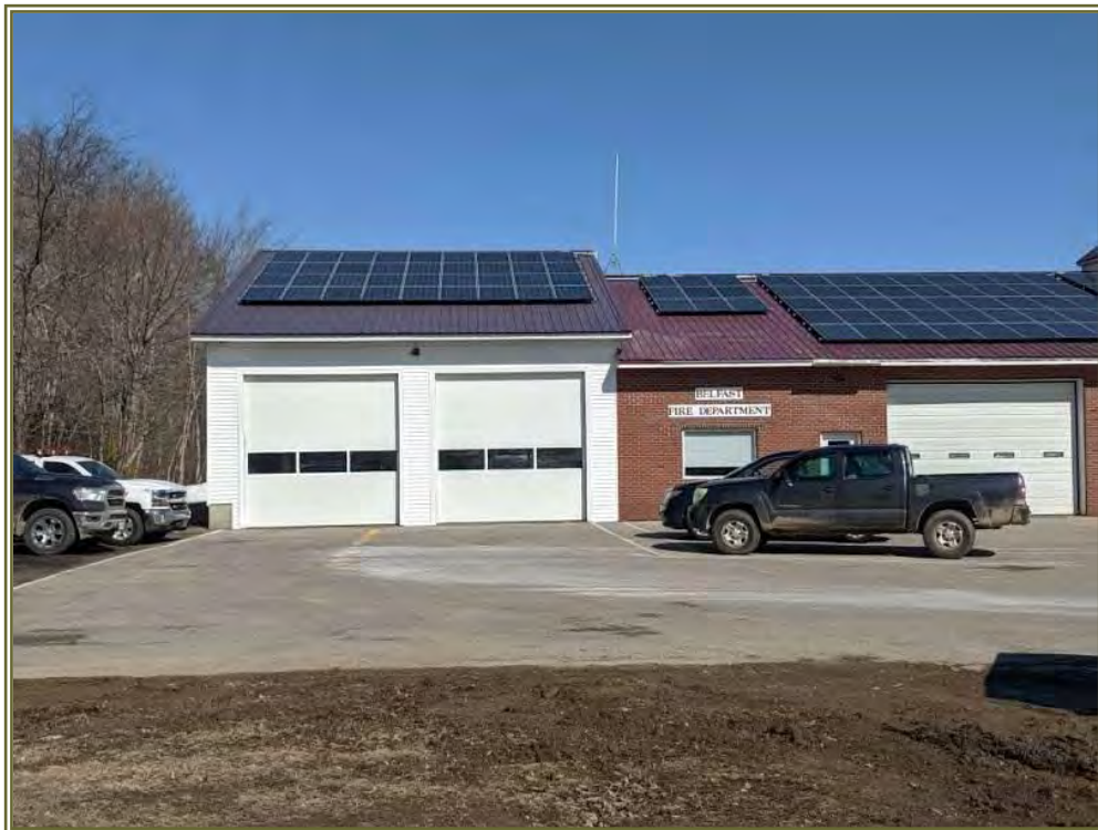
Front southwest side of Fire Station building with white sided addition looking north with parking on ground surface near drainage ditch
