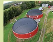
Microorganisms reproduce by feeding on the organic matter in the anaerobic digester, creating biogas.
