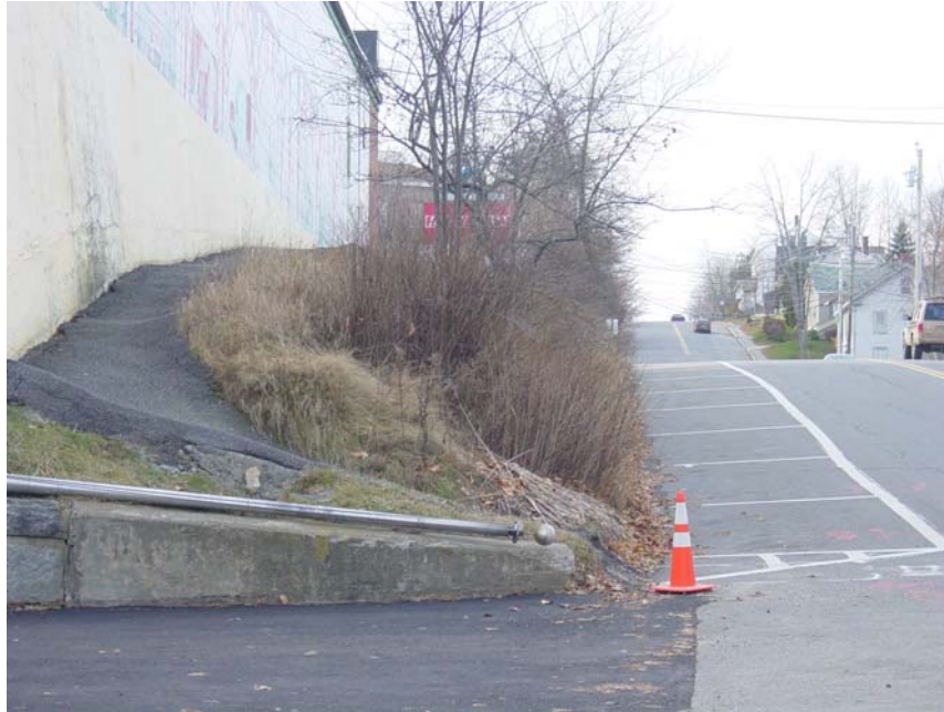
Figure 1. Parking and drainage swale next to Family Dollar
